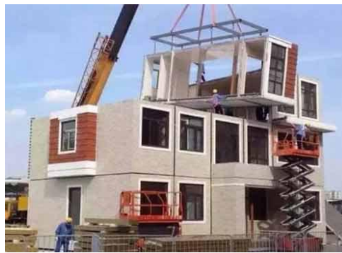
Figure 3 Assembly of modular buildings
