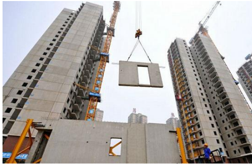
Figure 2 Assembly of prefabricated buildings
