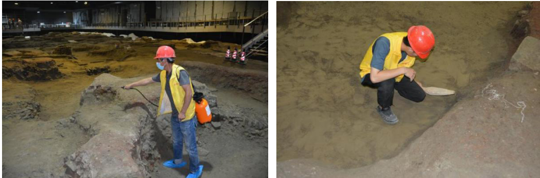
Figure 4: Spraying reinforcing materials and surface tamping
