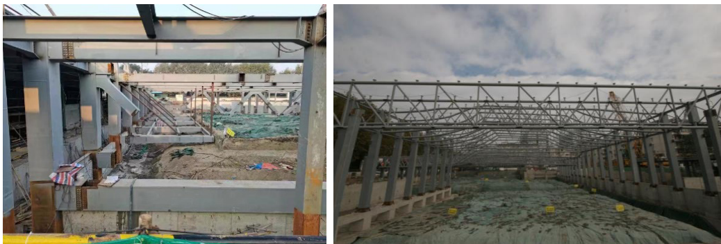
Figure 6: Non-ground-supported steel structural reinforcement system
