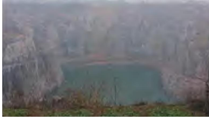
Figure 1 Panorama view of the deep foundation pit where the construction project is located
