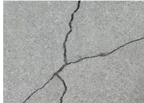
Horizontal crack and X-shaped crack
